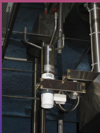
air flow monitoring to subway tunnels
